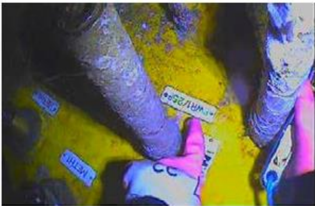
Initial attempt to remove correct Tronic unsuccessful
