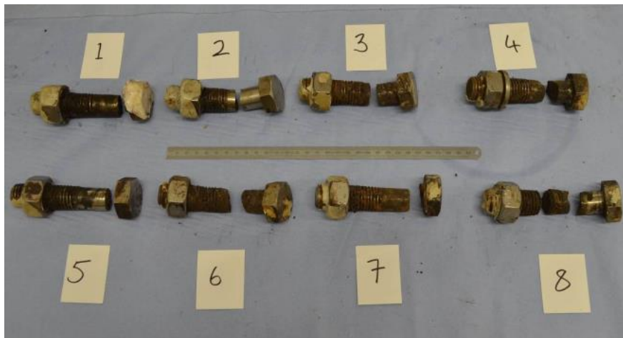
The condition of the severed bolts.
